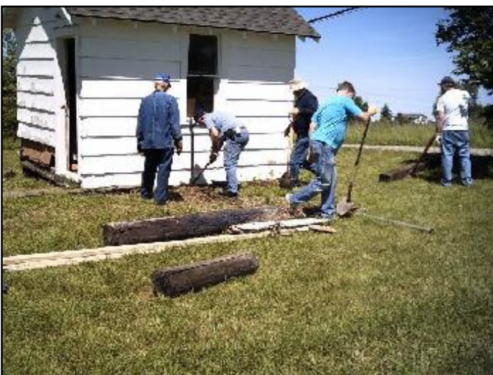
Starting to clean up the work site.
