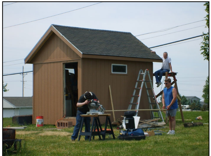
June 16, 2007: Damon, AB2UK, operates the chop saw while Doug, KA2WFT, steadies the board, and Dave, WA2TVT, awaits the trimmed board for installation on the north gable of the shack, now looking very sharp.
